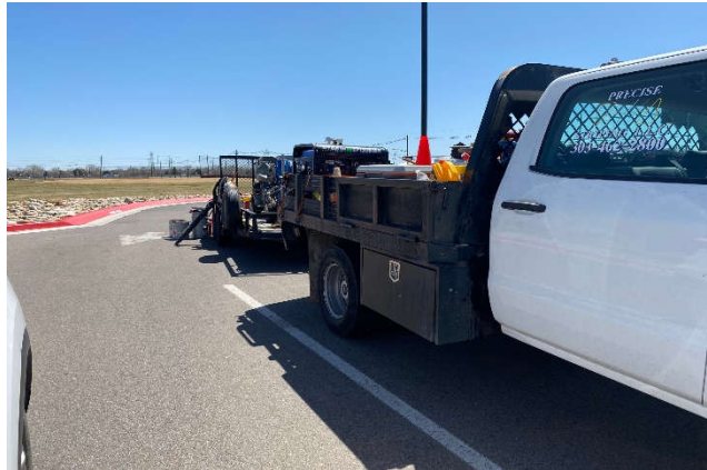
(Above)- Workers staged equipment for painting of fire lane curbs.
